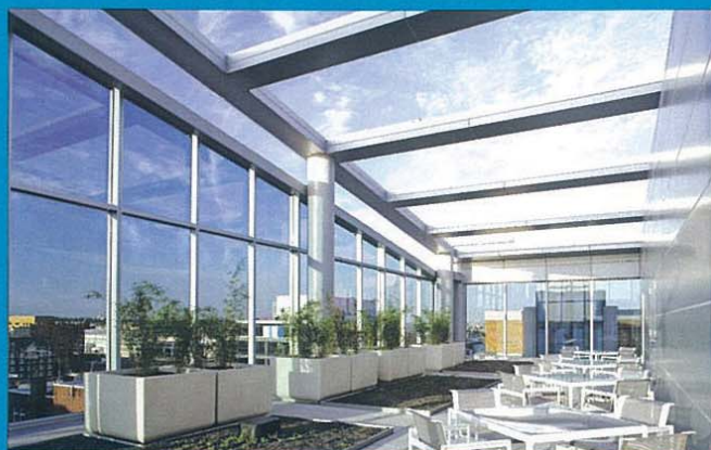
1050 K Street's green roof (shown in top left and bottom photos) captures rainwater and serves as an attractive function space with great city views.
